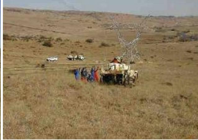
**Stringing pilot cable with pilot tractor**
